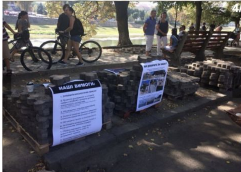
Uzhhorod Reconstruction of the central embankment
